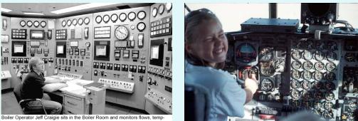
Boiler Operator Jeff Creigie sits in the Boiler Room and monitors flows, temperatures and pressures of the boilers and feed-water system. Photo by Ryan Solomon
